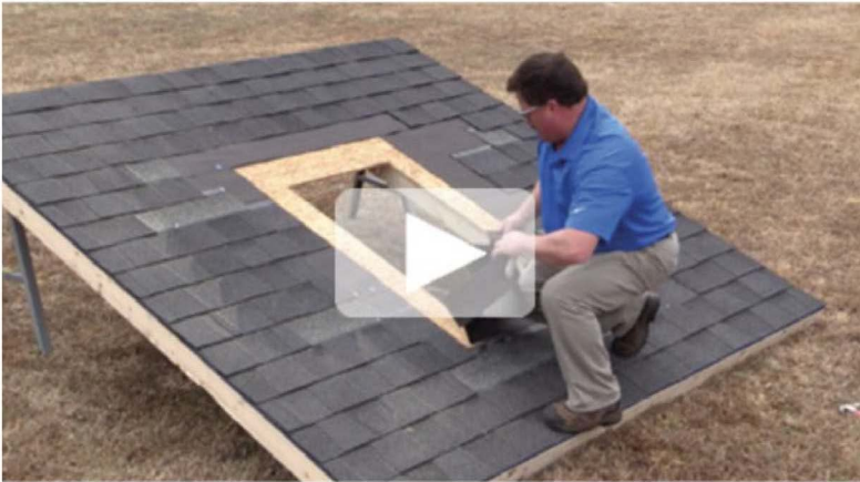
VELUX Install Video: Replacing Deck-Mount Skylights
