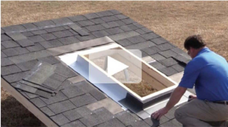
VELUX Install Video: Replacing Curb-Mount Skylights
